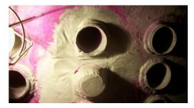
Fig. 4. Plugging of Bank Tubes of Boiler-II SGP NFL Naya Nangal.
